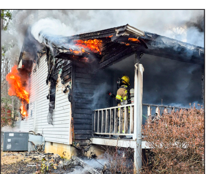
Union County Firefighters working hard to extinguish their first structure fire of the year on Forest Circle in northern Union County. Photo/Submitted
