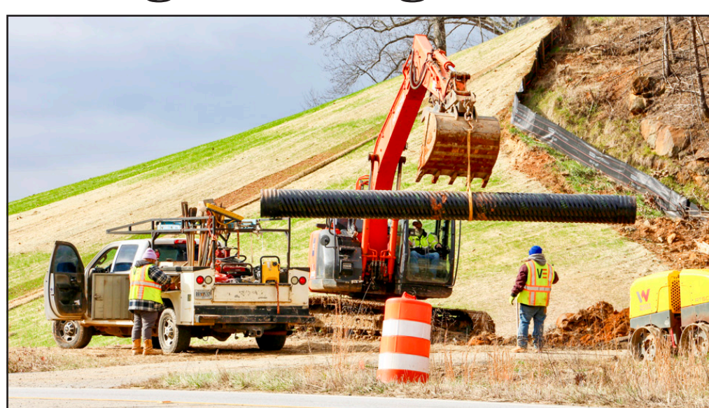
The Vertical Earth construction company is aiming to keep commuters happy as crews work to finish Phase II of GA 515 reconstruction as quickly as possible. Photo by Shawn Jarrard
